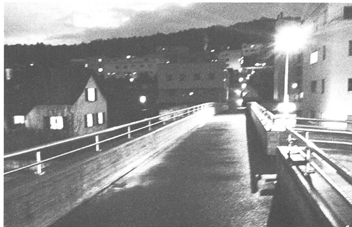
Wittenbachs Passerelle by night.
