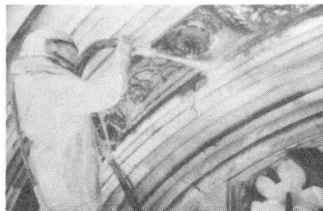
Fig.2 Blast Cleaning
