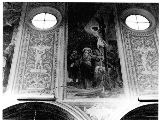
Fig. 5 - Fissures in the the wall defining the central nave.
