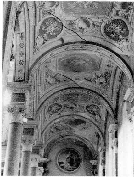
Fig. 3 - Fissures in the thin vaults of the side aisles.
