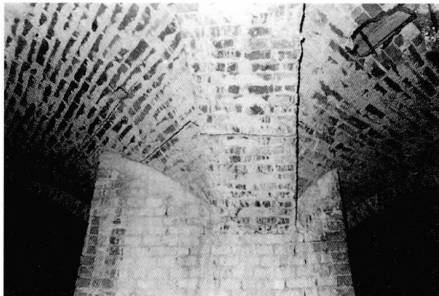
Fig. 4 - Fissures in the the 12 cm thick vaults on the underground level.
