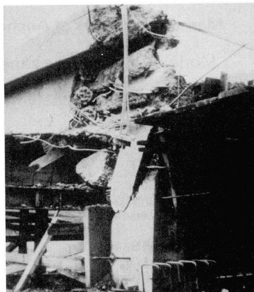
Figure 1: Failure of an Anchorage Zone in a Pedestrian Bridge during Construction
