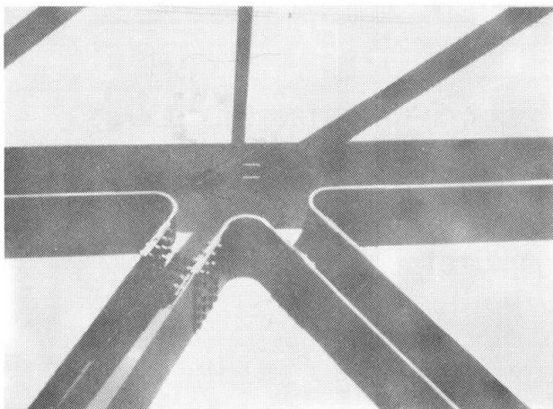
FIGURE 2 : An example of a fatigue-resistant detail.
