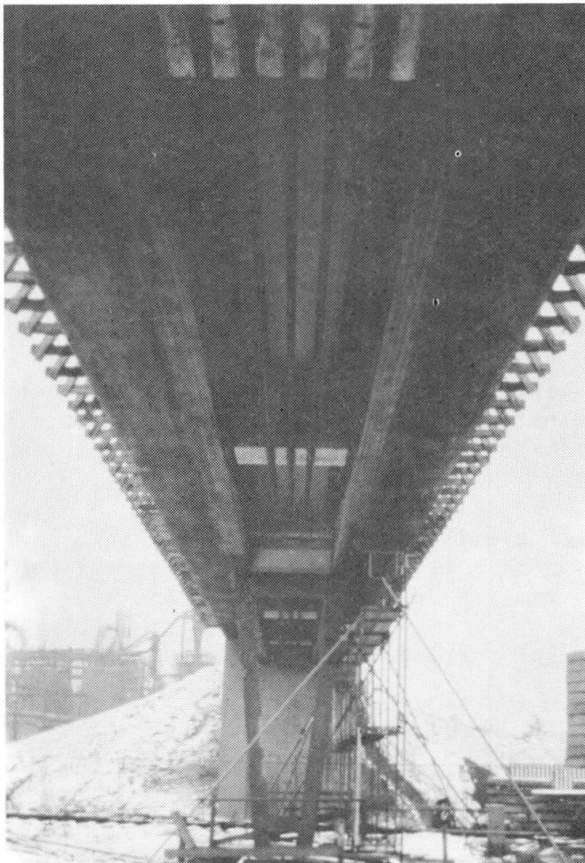
Fig. 2 External application of the prestressing tendons
