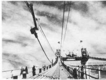
Erection of cable
