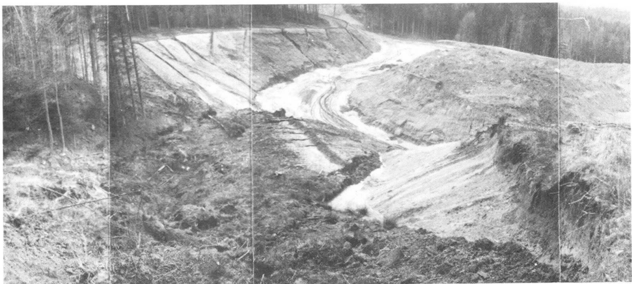
Figure 7 A Rock Mass of 29,000 m 3 Glides Off.
