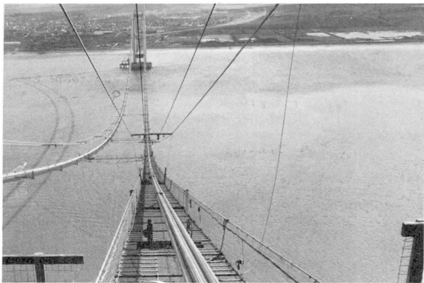
Mainspan cable part way through spinning process.
