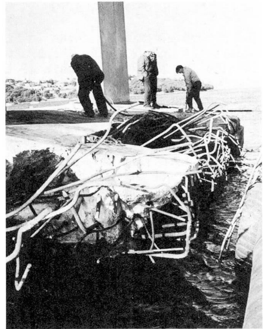
Fig. 5 Damage to Pile Cap 20
