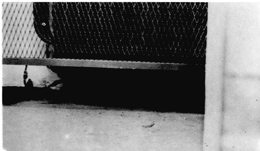
Fig 3. The transformer inside the cabin has moved during the earthquake; one of the back wheels fell into the oil drainage well.
