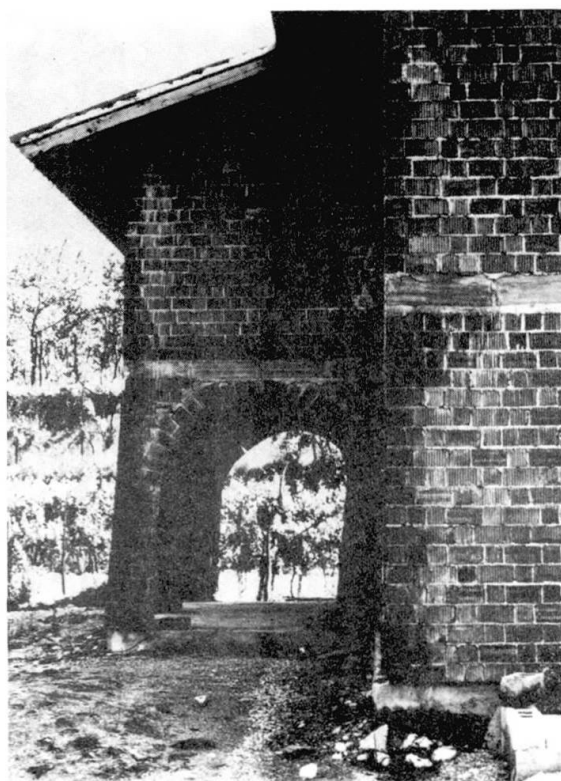
Fig. 9 Gemona; the building moved back and forth on the concrete base.
