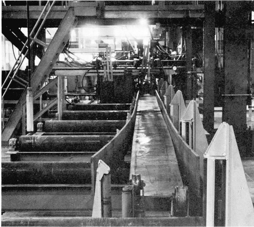
Fig. 8 Entering First Welding Unit (Courtesy Inland Steel Company)
