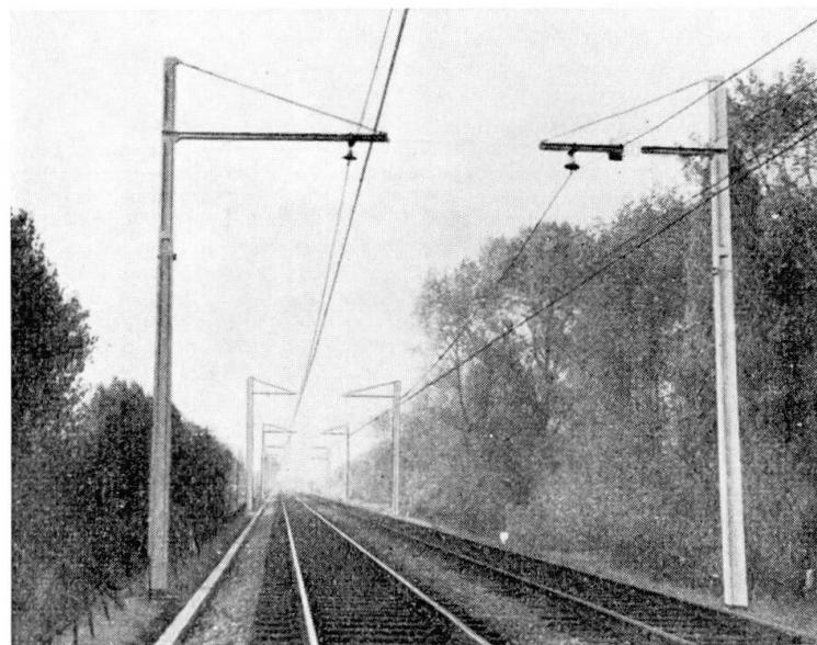
Fig. 1. Prestressed Concrete Cantilever Masts near Southend (England).
