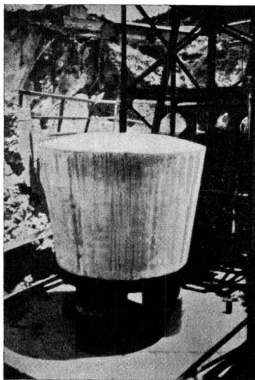
Fig. 7. Concrete head of anchoring tie on three hydraulic jacks.
